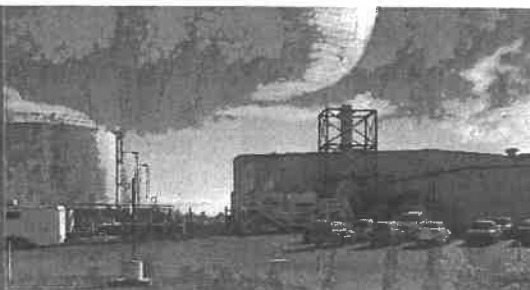
Outside the 200 East Area Effluent Treatment Facility
